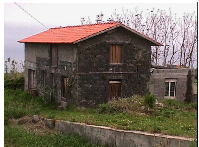
Fig. 8. Dwelling with external walls in stone and in concrete blocks.
